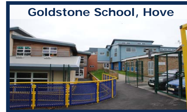
Goldstone School, Hove Description: Extension & Alterations Client: Brighton and Hove City Council Value: £ 2,770,000
